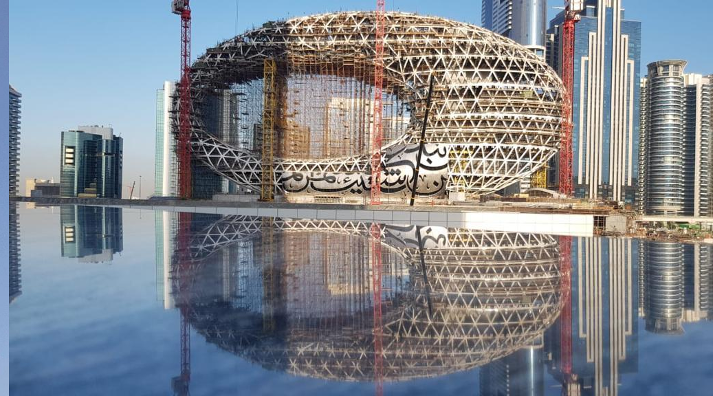
Tower cranes: 2 x WOLFF 355B & 1 x WOLFF 8033.20
