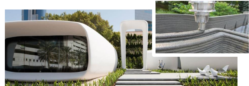
The world's first fully functional 3D-printed building in Dubai
